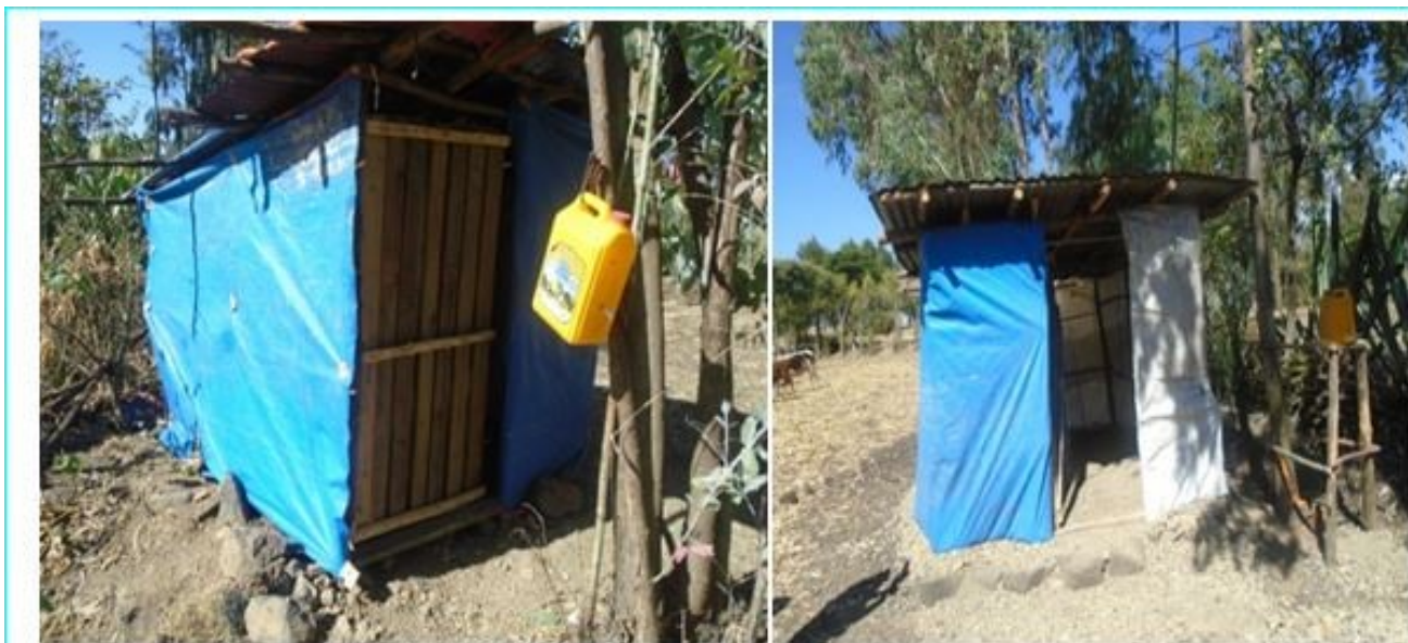
Improved household pit latrines
